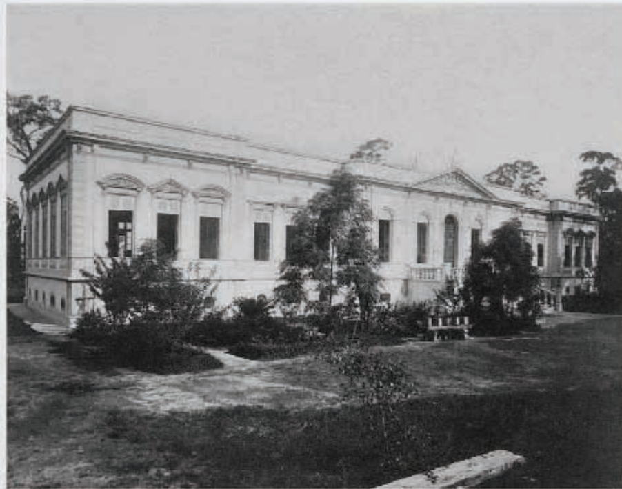
HOSPITAL DOMINGOS FREIRE
